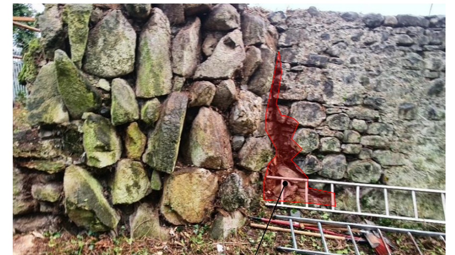
Outer face of North-West Flanking Wall
