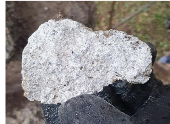
Existing lime-rich mortar on site
