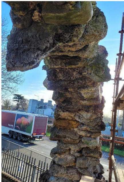
Figure 3 – Underside of arch
