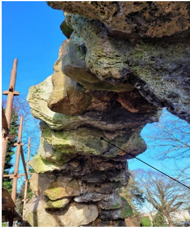
Underside of North-West side of Arch
