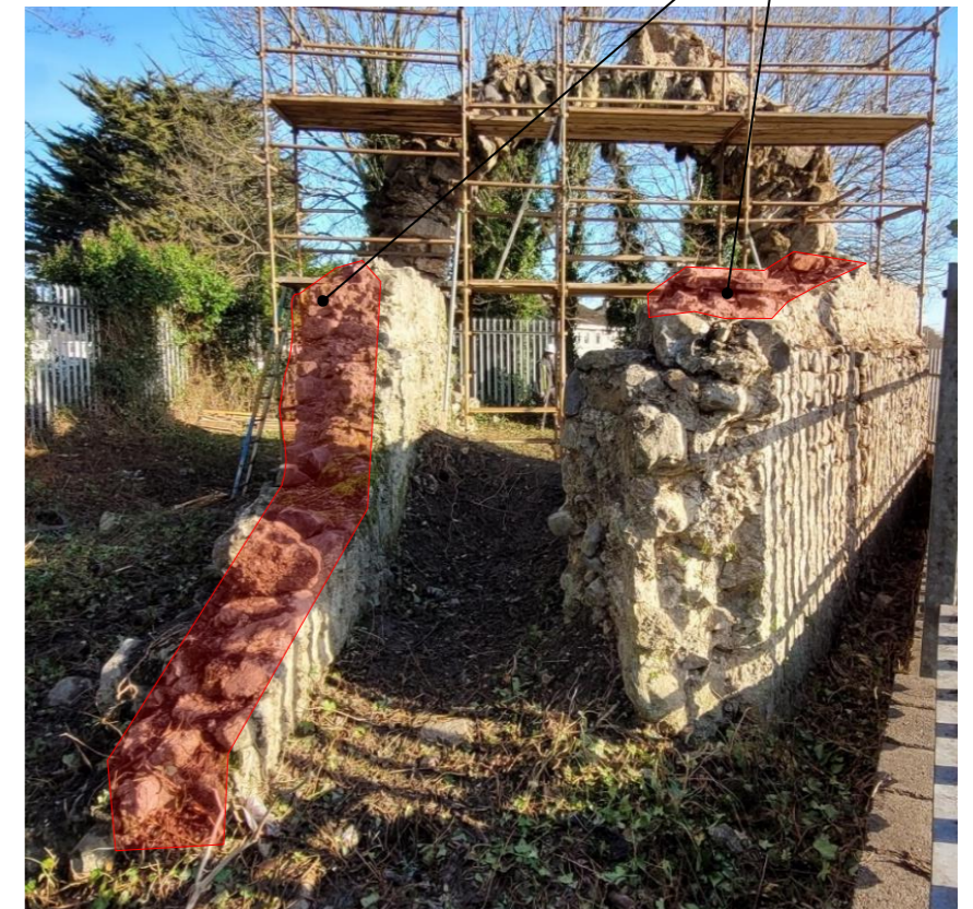
Arch and Flanking Walls viewed from South-West
