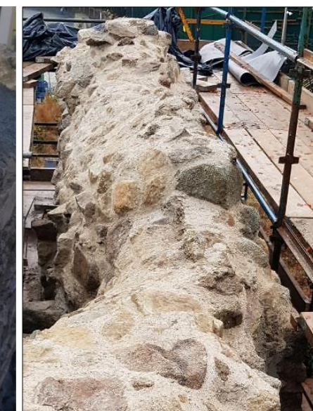
Sample of regularised (left) and rough-raked (right) wall top finish
