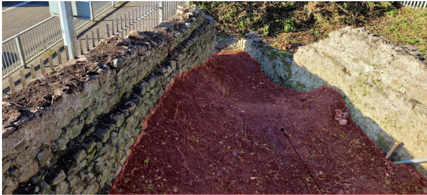
Area between Flanking Walls viewed from the top of the Arch
