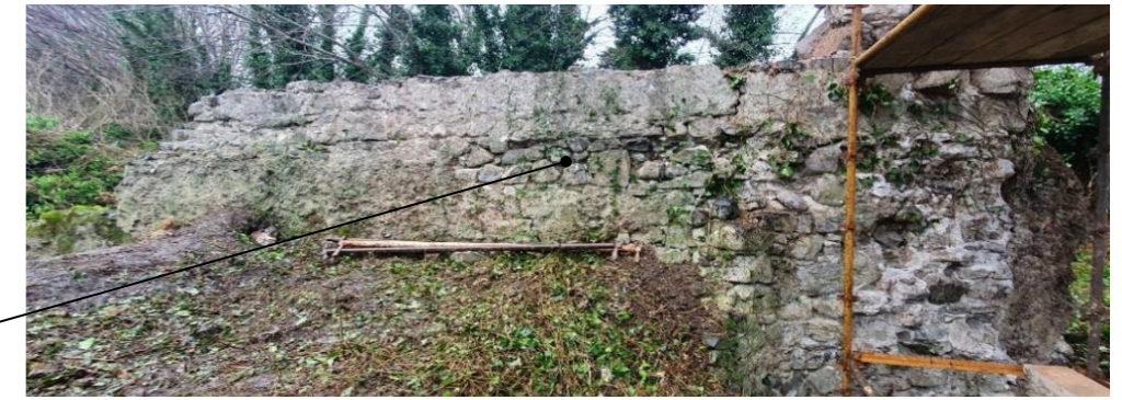
Inner face of North-West Flanking Wall
