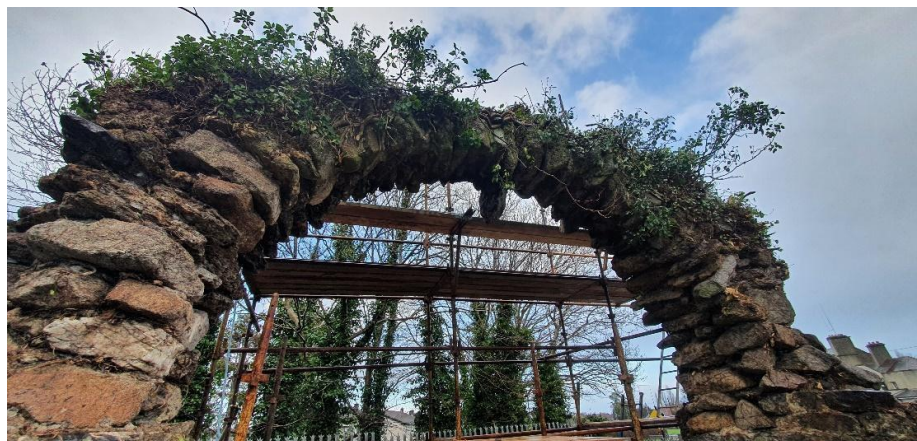
Figure 6 – Arch during vegetation removal
