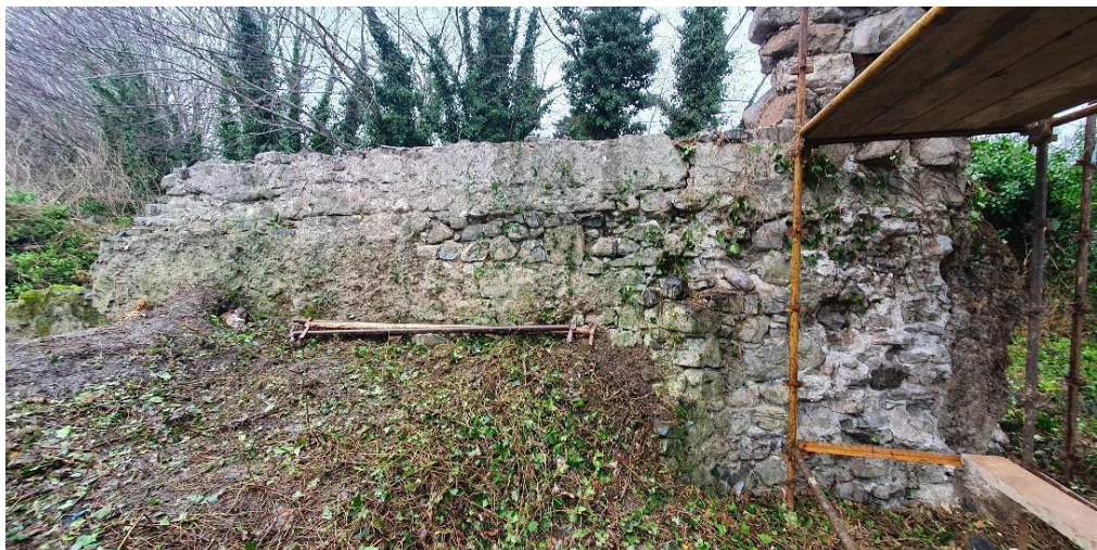
Figure 13 – Inner face of northwest flanking wall
