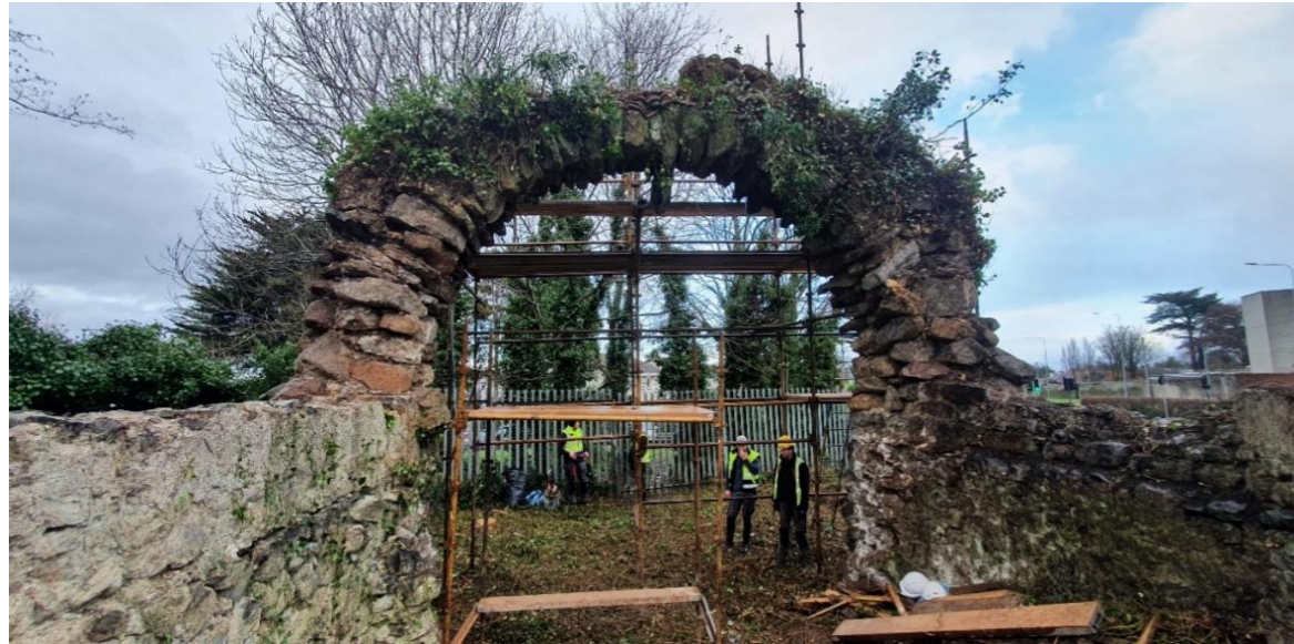
Arch during vegetation removal viewed from South-West
