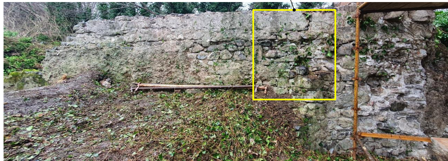
Inner face of North-West Flanking Wall
