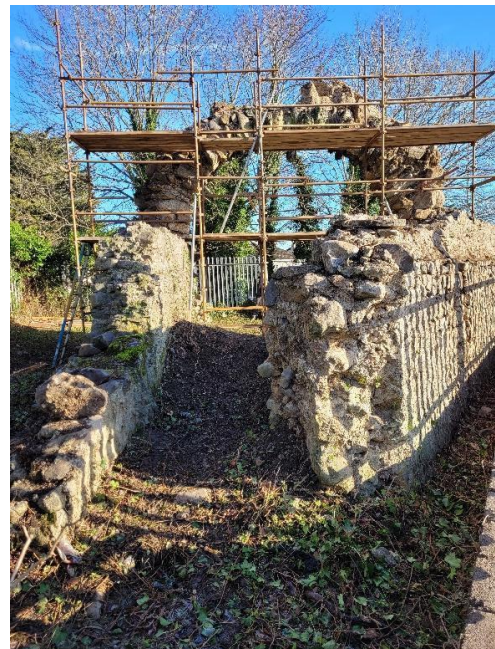
Figure 9 – Arch and flank walls after vegetation removal
