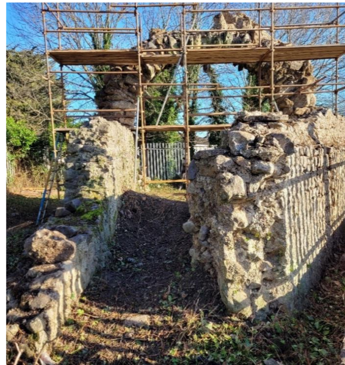
Arch and Flanking Walls viewed from South-West
