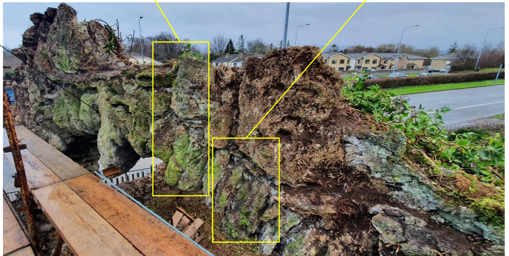
Top of North-East side of the Arch
