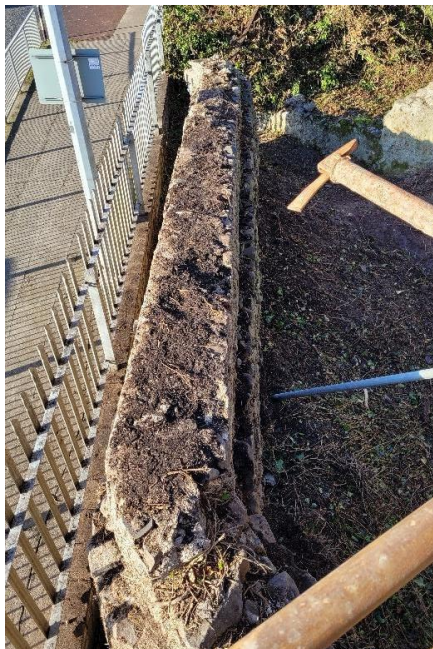
Figure 8 – Top of southeast flanking wall
