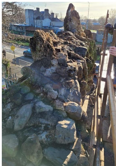
Figure 7 – Top of arch after vegetation removal
