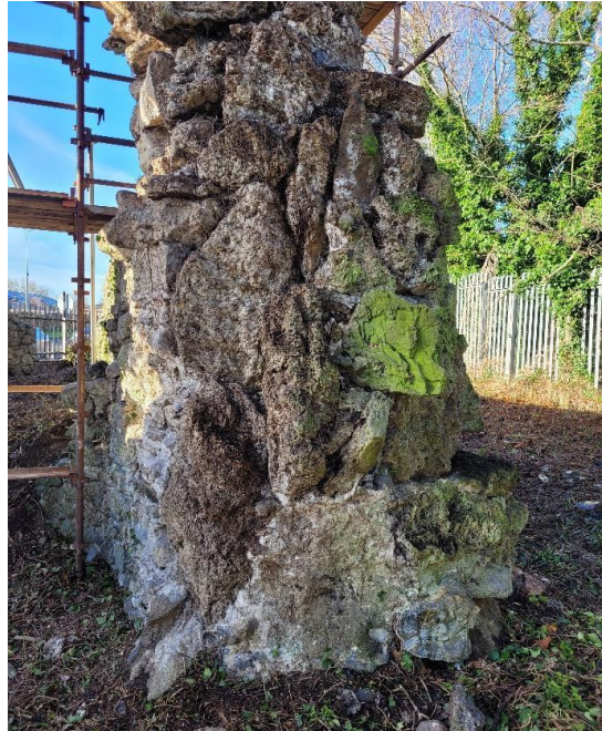
Figure 17 – Base of arch with various stone types and algae/lichen-stained stone
