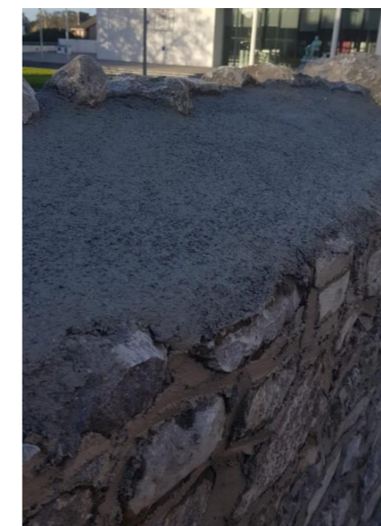
Sample of regularised (left) and rough-raked (right) wall top finish
